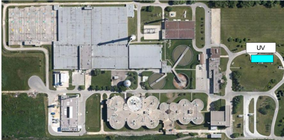
Figure 2.28 UV Disinfection Facility
